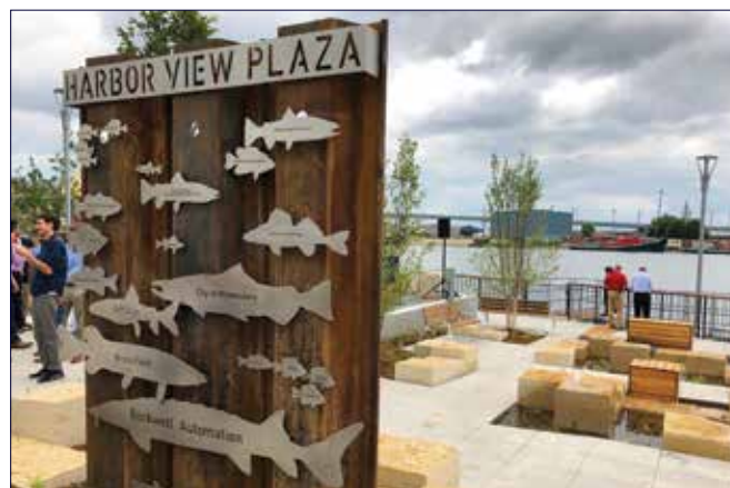
Harbor District, Inc. constructed and partially funded the newly-opened Harbor View Plaza to provide public park space and water access along Milwaukee's inner harbor. (credit: Bobby Tanzilo - OnMilwaukee.com)
